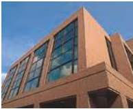
D Building No.2
