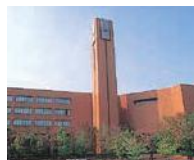
M Building No.17
