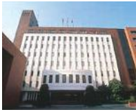
A Main Building
