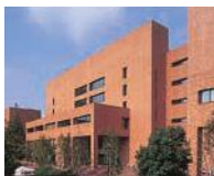
L Building No.16
